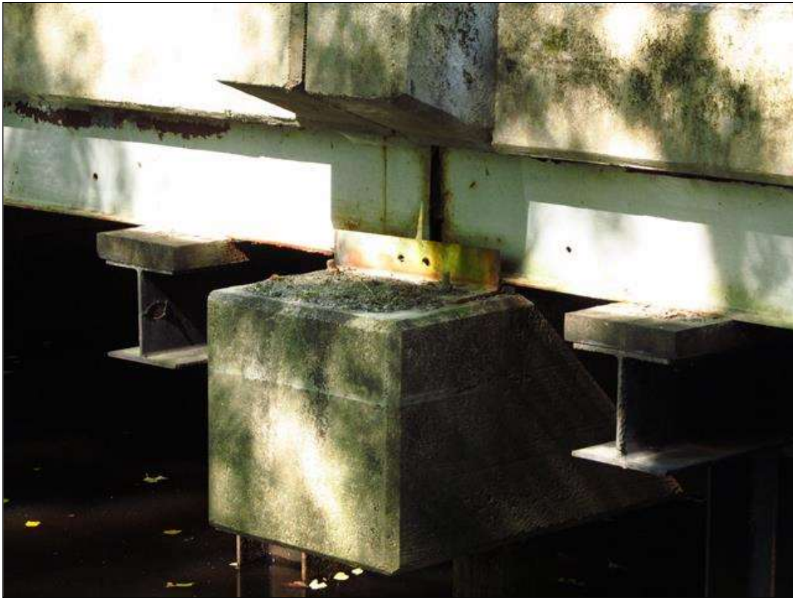
Superstructure over End of cap
