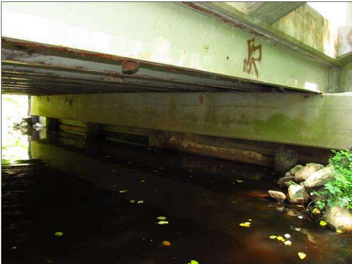
End Bent 2 overview
