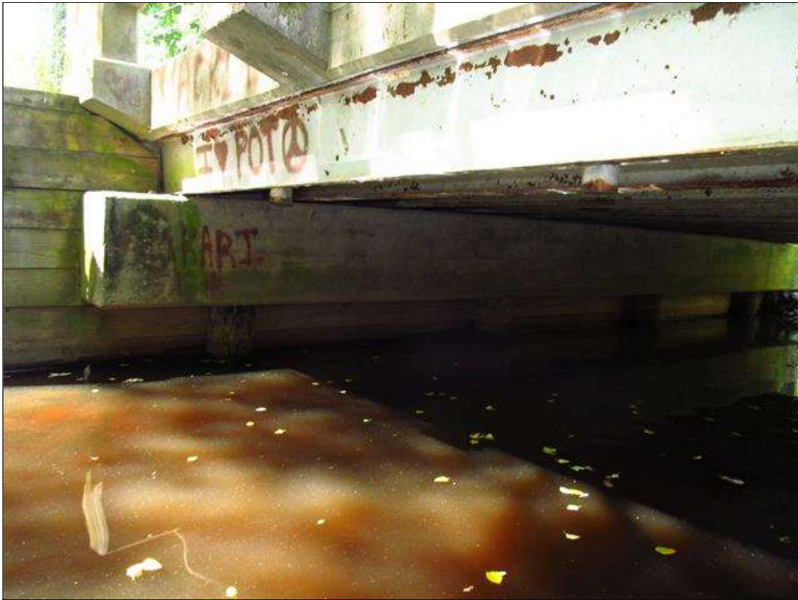
End Bent 1 overview
