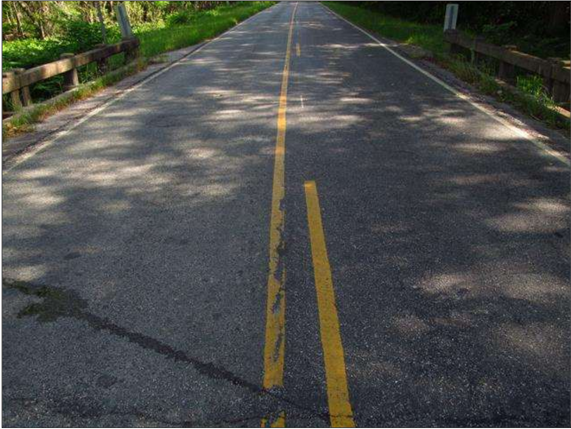
Asphalt wearing surface overview
