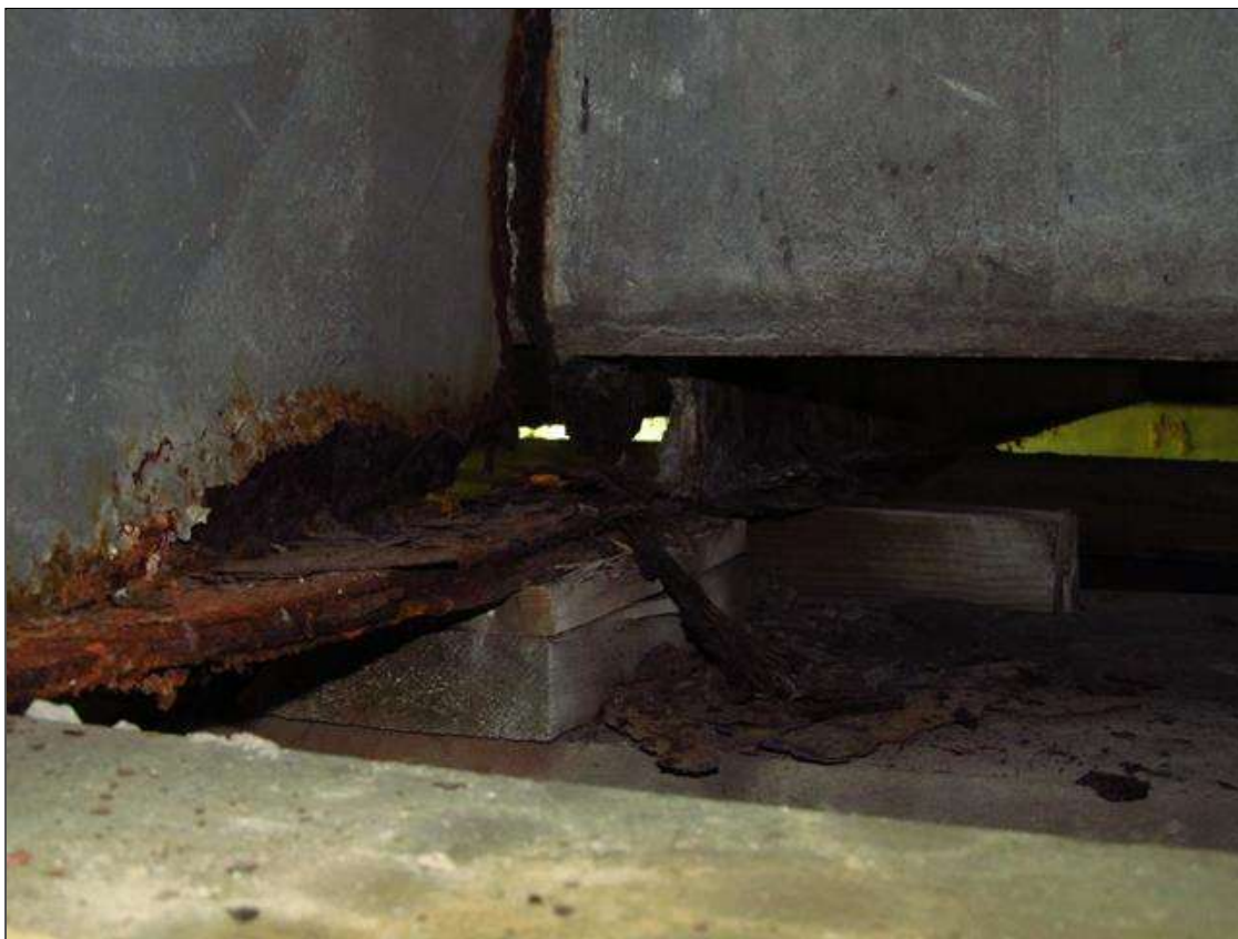
Section loss in the end of Beam 2 in Span 1 over Bent 1 - other beams similar throughout structure
