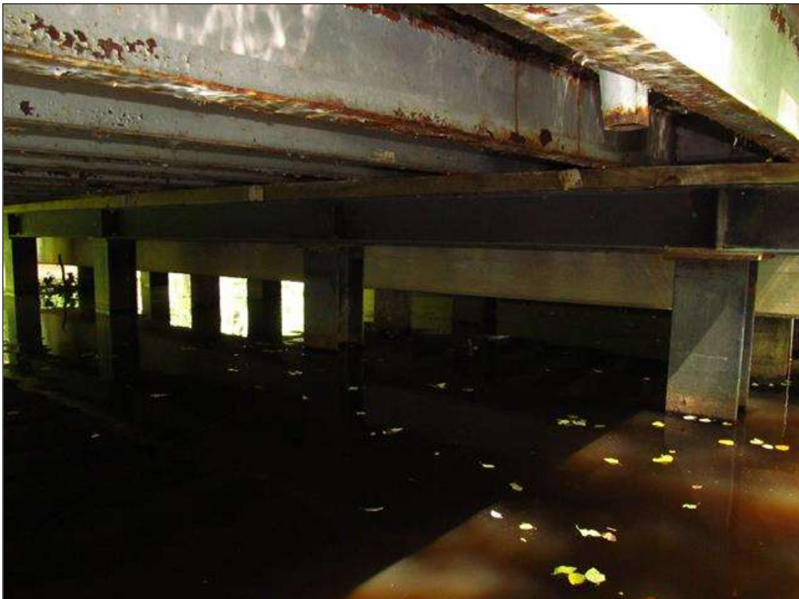
Bent 1 Span 1 side
