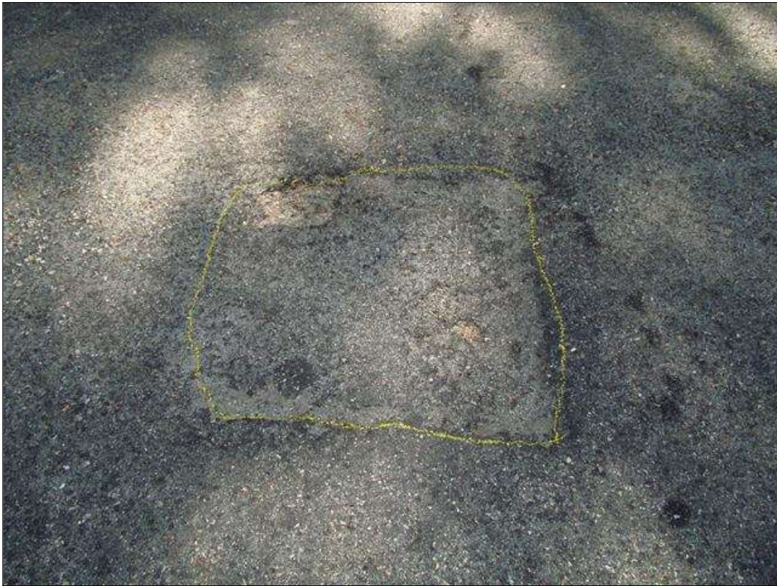
4 square feet of asphalt settled in the Southbound lane of Span 2
