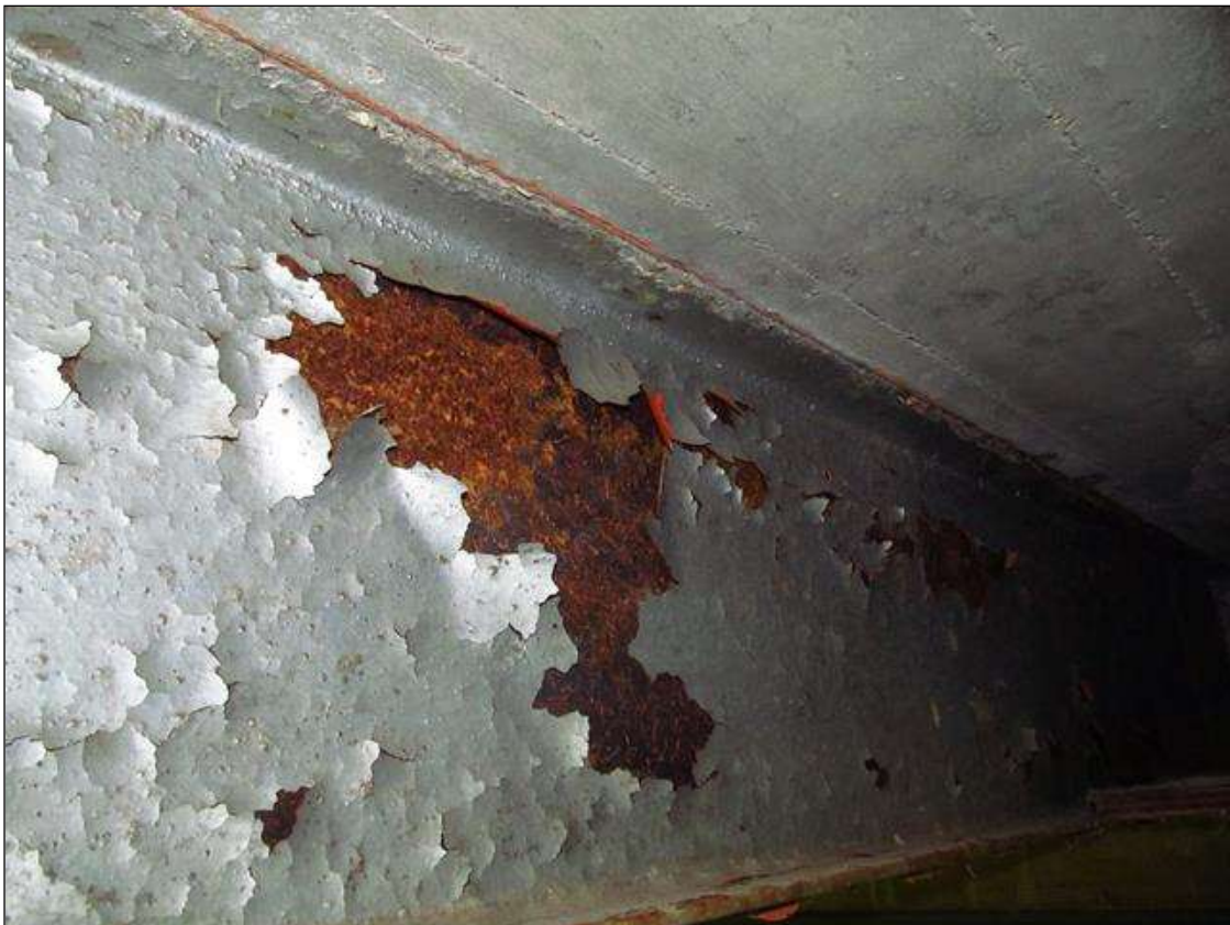
Areas of failed protective coating throughout structure
