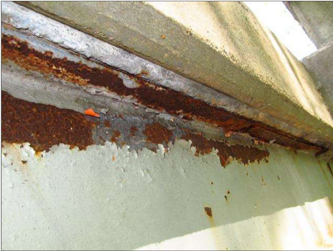
Corrosion along beam flanges and webs throughout structure
