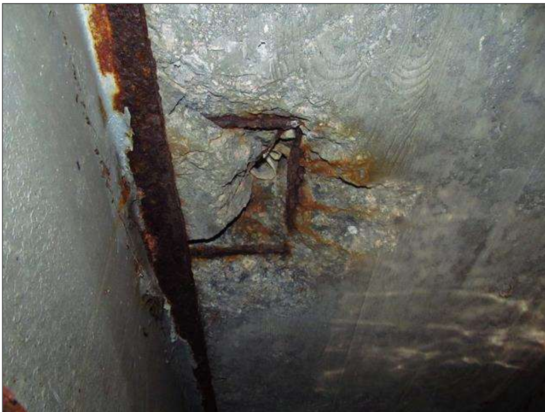
Spalling with Exposed rebar in Bottom of deck where crutch bents were added
